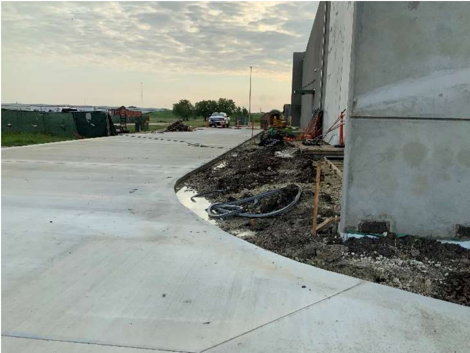
Fire Lane being extended
