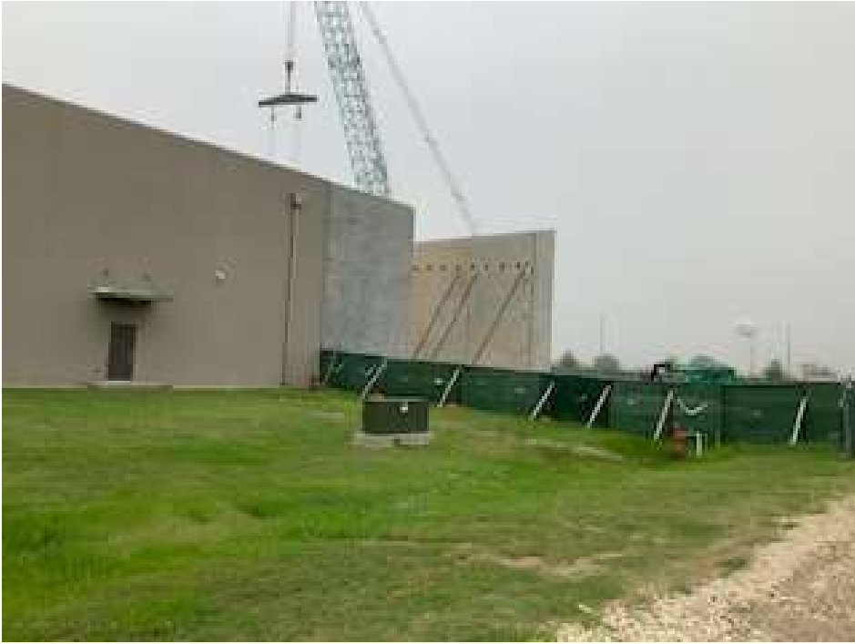
Walls going up
