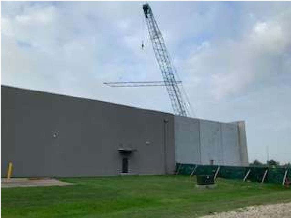
Roof going on
