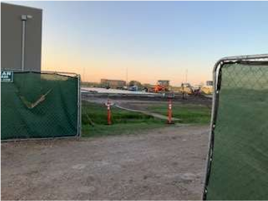
Floor being poured
